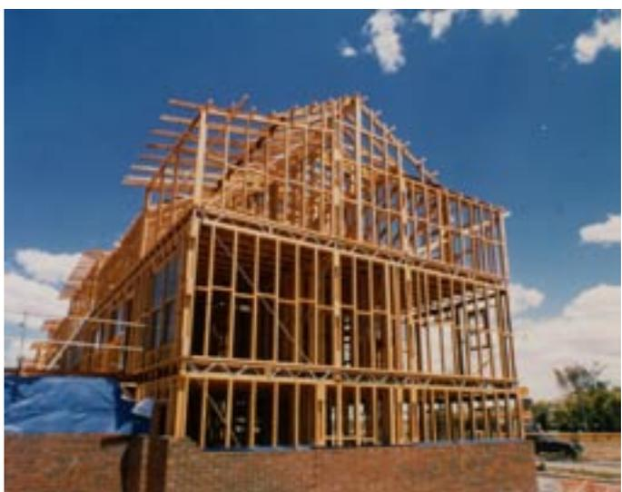
*Multi-storey constructions are less likely to be located in bushfire-prone areas. Even so, fire-resistant timber can still help to reduce the effects of 'normal' fires. By building with fire-rated timber, protected by appropriate lining materials, it is possible to prevent fires from spreading.*
