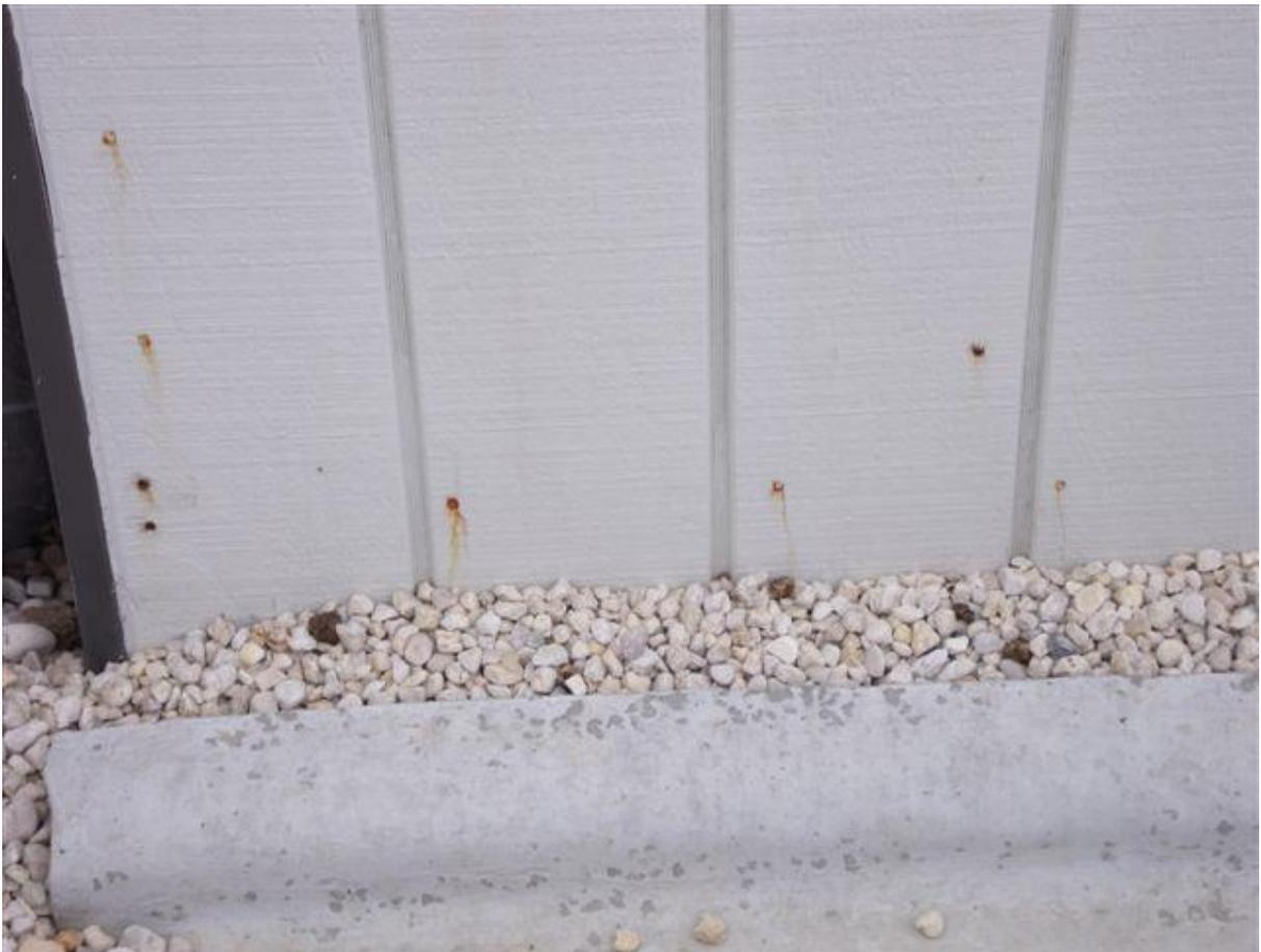
**FIGURE ONE: Corroded Fasteners in Preservative Treated Plywood Cladding**
