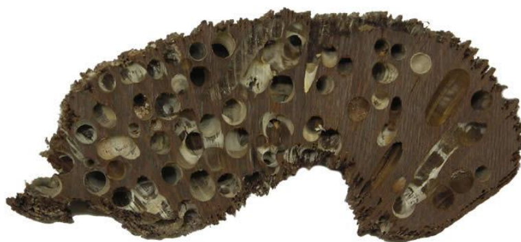
Marine borer damage to a hardwood pylon
