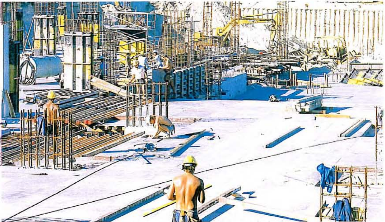
Soffit formwork at the stage 1 phase of the construction cycle.
