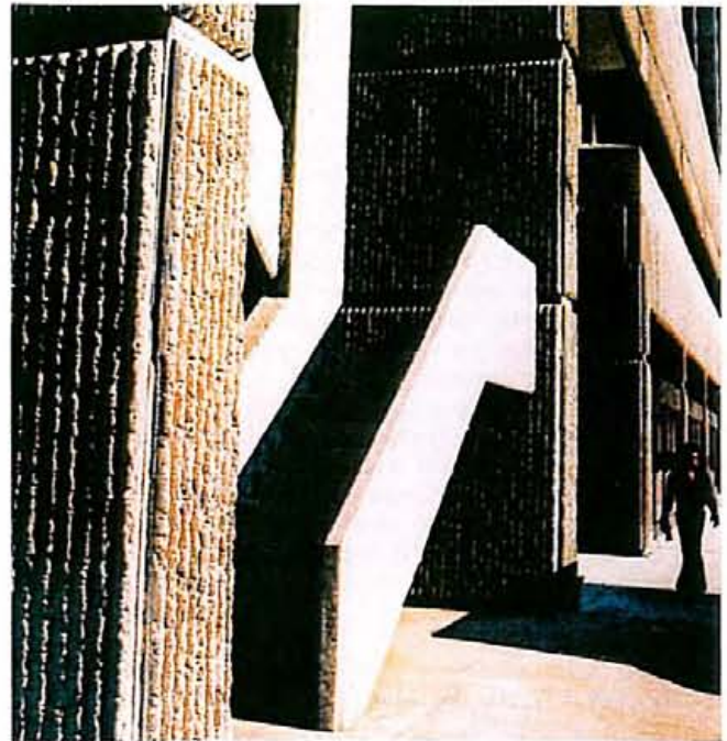
An architectural concrete surface typifying the use of rope liners.
