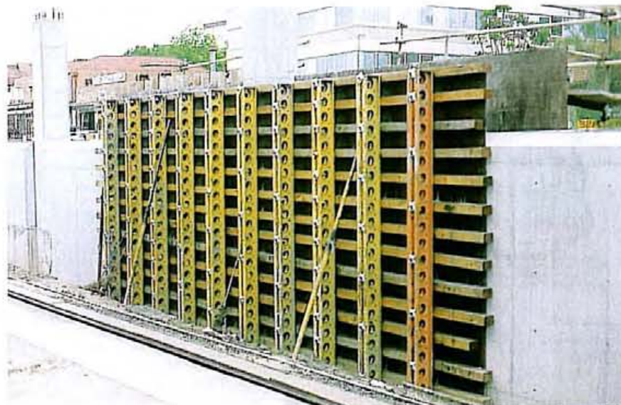
Stiffening the bottom edge of the form.
