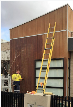
STAINING: Stain in the same direction that the boards run - vertical for vertical cladding.
