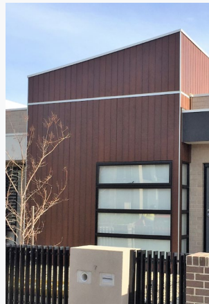
COMPLETE: After 3 coats the timber is restored and is now UV protected.
