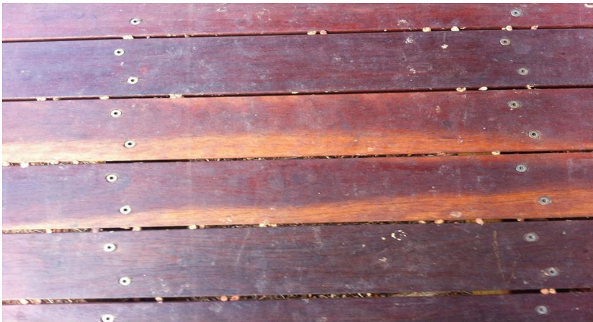
Figure 6. Ironbark decking with untreated sapwood
