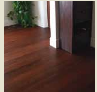
Colour darkens as the temperature in the process is increased
