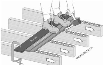
As the leading edge of the board engages with the leading teeth, the trailing edge will move clear of the trailing teeth on the other side of the board, allowing the board to sit flat on the base of the clip. Work towards either end of the board to fully engage the leading edge into the clip.
